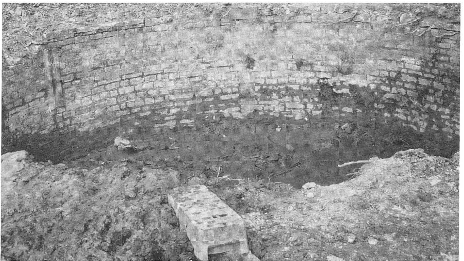
12: Remains of the larger of two gasometer pits
