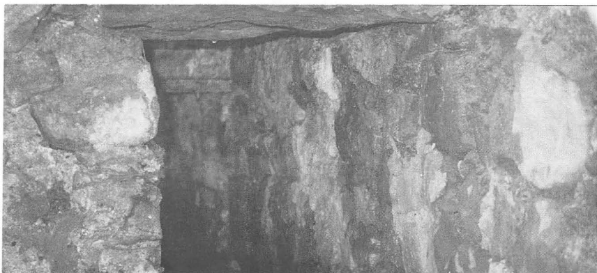
14. Culvert , sluice down stream leading under road, to River Chew
