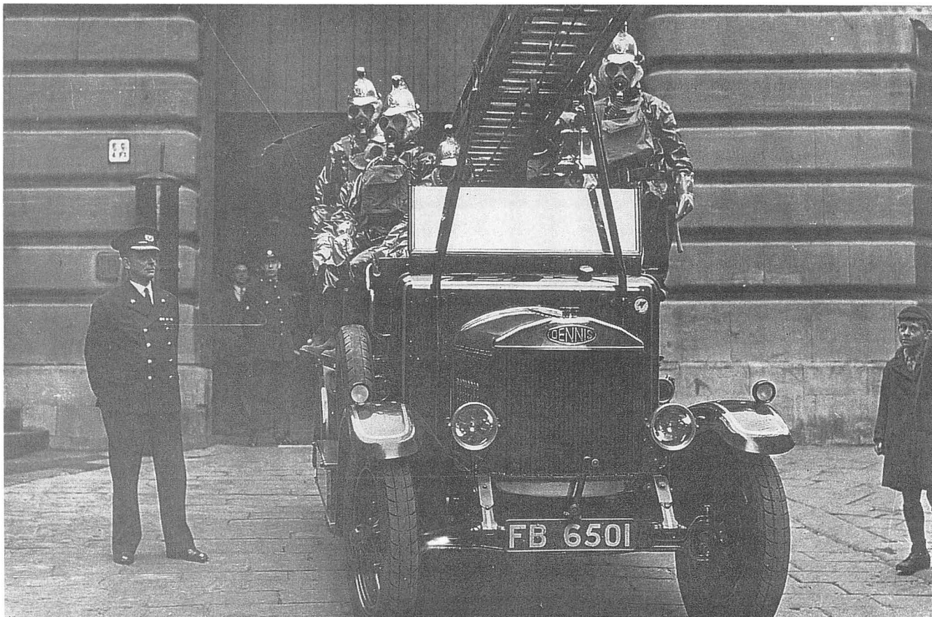
3. Chief Officer James Hurst (standing left) with members of Bath Fire Brigade in 1938. CO Hurst found emergency water supplies in villages such as Corston, Kelston and Newton St Loe to be woefully inadequate
