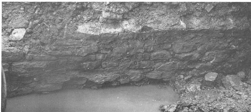
15. West wall of culvert, Gas Works, Dapps Hill
